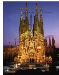
Lighting enclave and monumental sets.
