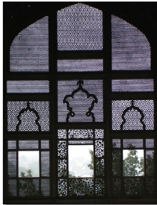
Plate 9. Central largest white marble jālī screen of Shish Mahal of 1631-34 at the Lahore Fort. (8" x 10") Source: Photograph by the author.
