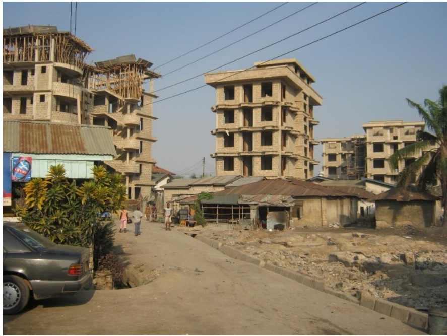
Figure 6: Shengena access road that is transforming into Commercial Street
